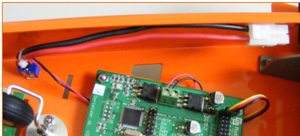
Figure 5.0 – Wiring Harness power leads properly connected to Serializer
